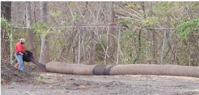
Figure 7. Installing a 24" Filtrexx SiltSox. Photo by Cary Oshins
